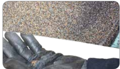
The steel shingle, including lock seam, is cut in an easy, steady motion. The shearing action has a "wiping" effect on the shingle's zinc coating that seals cut edge to resist rust.
